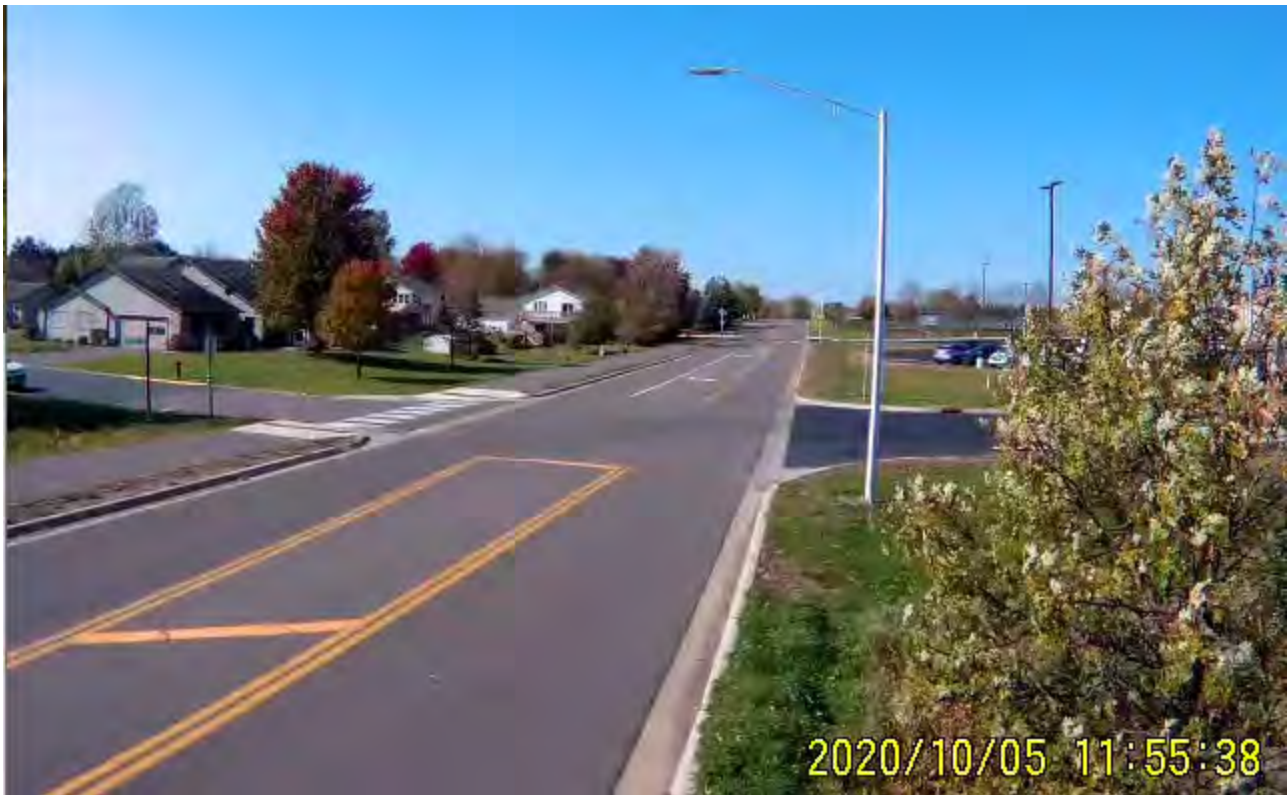
Looking westerly along 9 th Street at the Sunset Lane intersection and entrance to the elementary school. The trail and the eastbound left turn lane to the school are apparent. The pedestrian crossing at Village Green Lane is visible in the distance.
