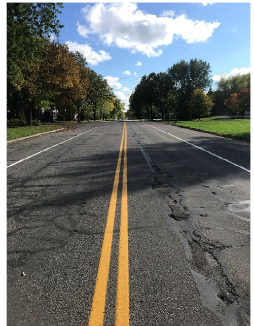
Existing pavement condition south of Maple Ave
