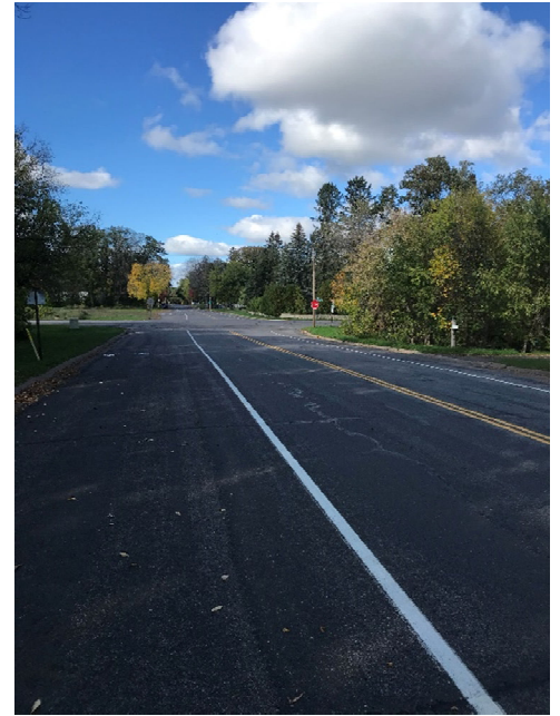
Current on-street trail
