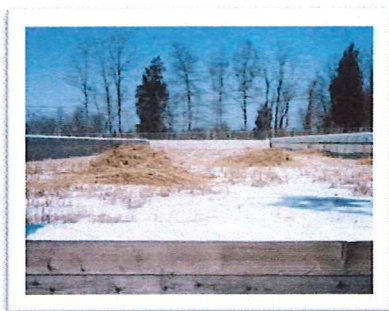
Harvested reeds prior to removal from the Reed Bed (cutting method)
